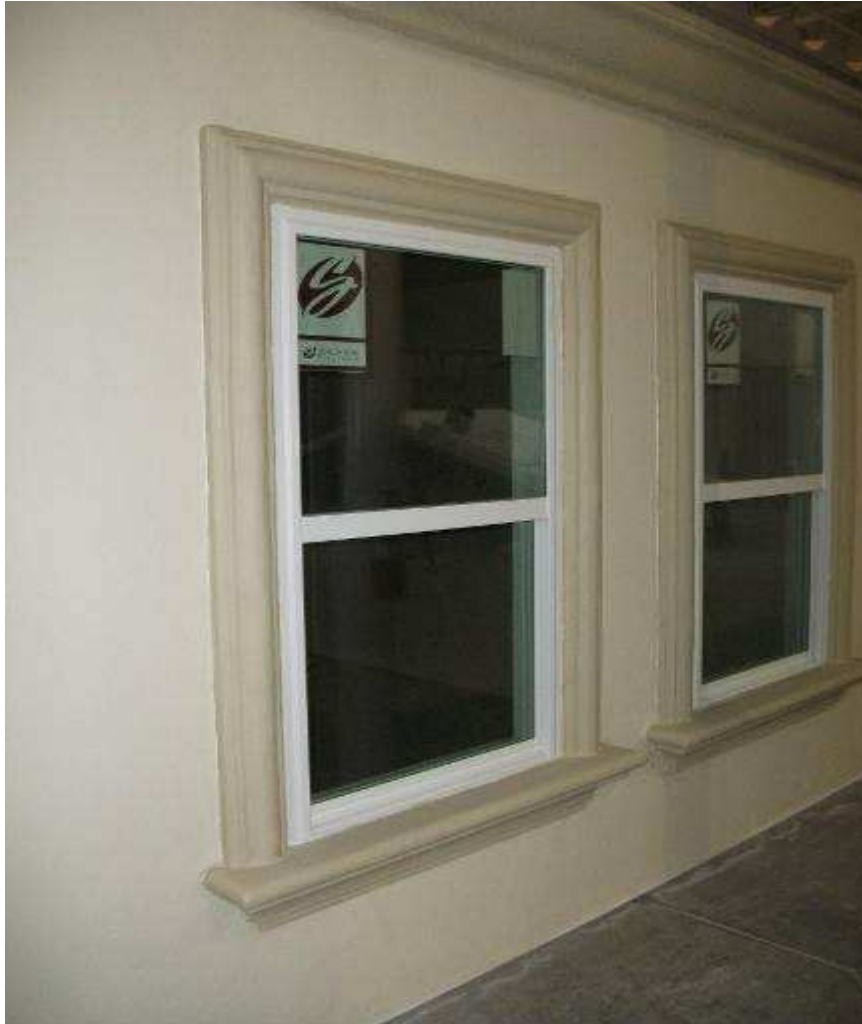
Window and Door trims cut from EPS foam are covered with StuccoMax
