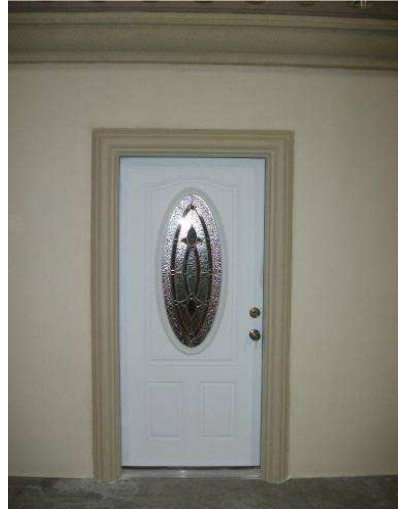
Window and Door trims cut from EPS foam are covered with StuccoMax
