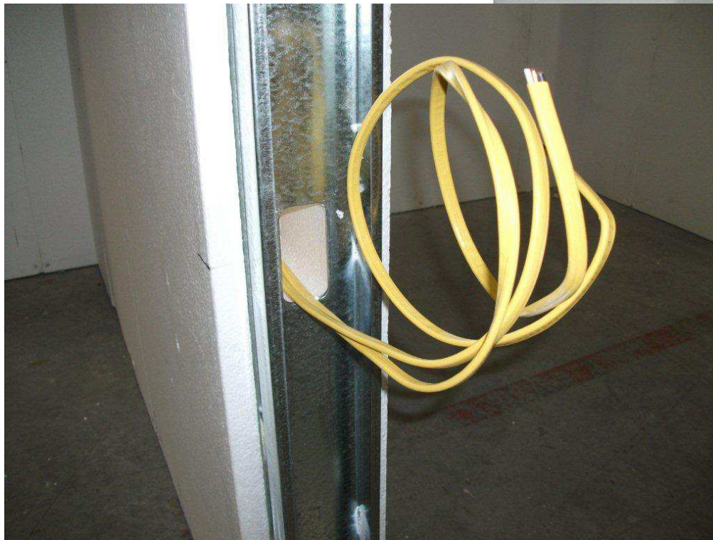
Electrical wiring inside chase
