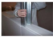
Insert studs and panel to panel inline connectors. Connectors fit into the bottom track and fit flush with the top of the panels.
